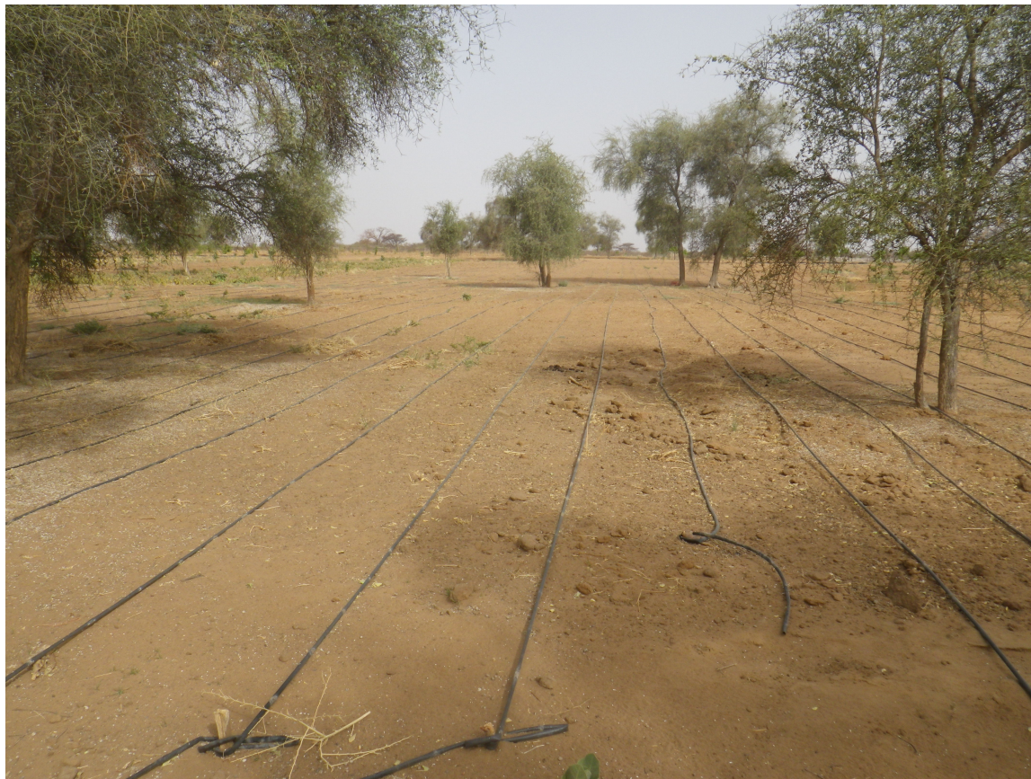
Figure 5.4: Drip irrigation system in the community garden of Widou Thiengoly. The irrigation system did not work during the study period. Photo taken June 2013.
